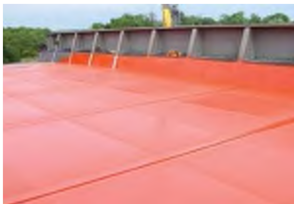
Bridge Deck Waterproofing
