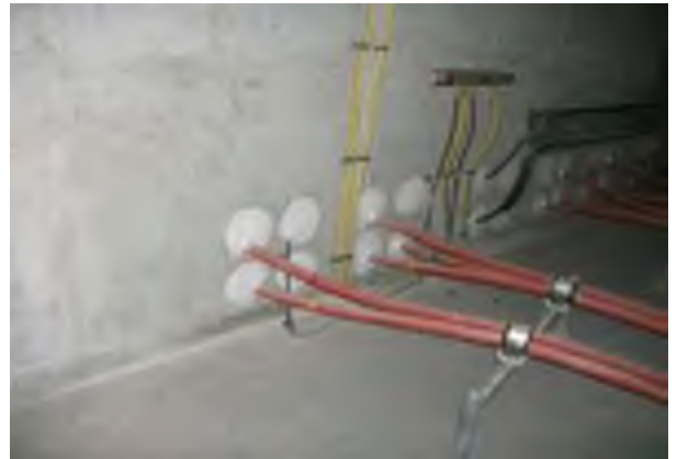
Sealant for Cables
