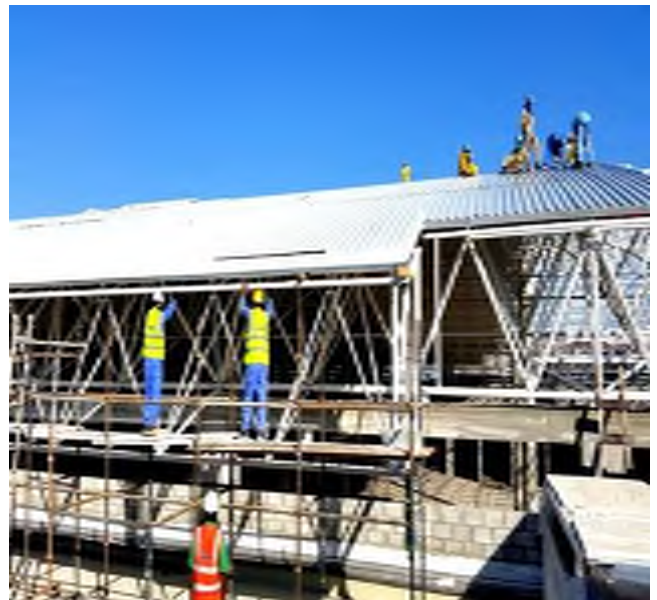
Steel Structure Cladding
