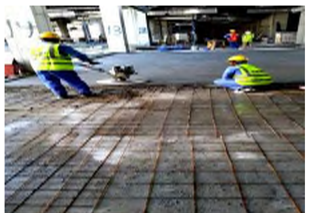
Flooring Repair and Screeding
