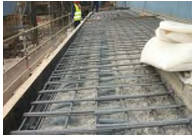
Slab Concrete Repair
